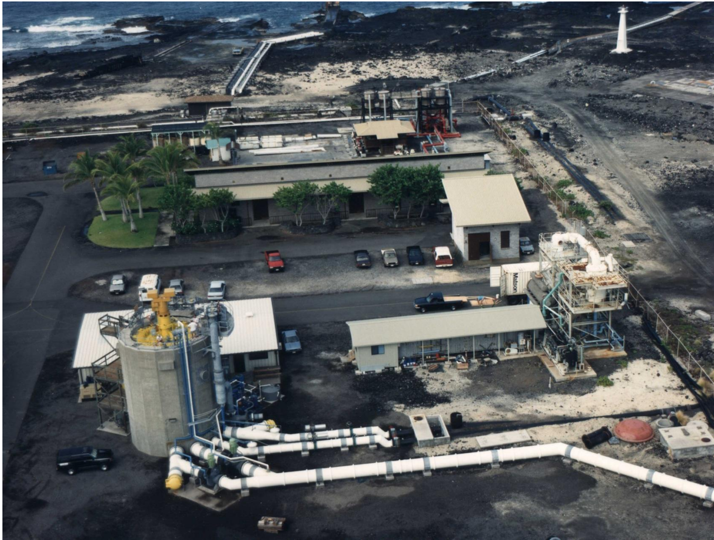
210kW OC-OTEC Experimental Plant (1993-1998) in Hawaii
