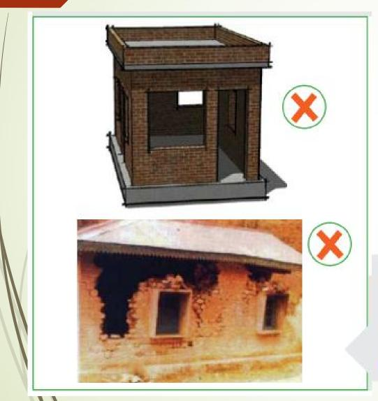
Openings are the most Vulnerable part in a building. Large shear forces get accumulated around openings and therefore, edges of the openings should be specifically strengthened.
