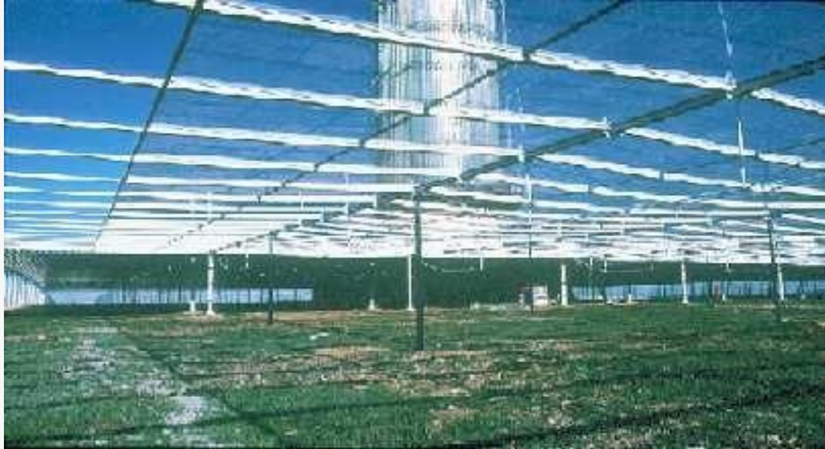
Fig. The glazed collector roof of Solar Chimney
