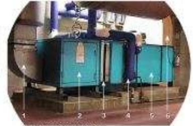
AHU COMPONENT 1 - Supply duct 2 - Fan compartment 3 - Flexible connection 4 - Heating and/or cooling coil 5 - Filter compartment 6 - Return and fresh air duct
