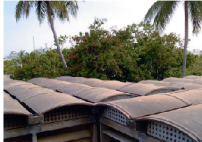
Fig. 11 Precast concrete roof, gutter and sill used in Okavango Paddock
