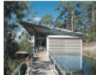
Fig.29 Application of Steel in Building
