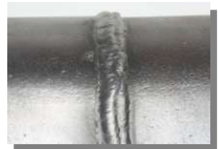
Final weld after several beads are made
