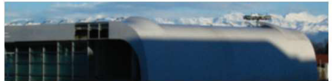
The newly opened Sheraton Hotel in Milan features a dramatic design achieved through the use of exterior cladding made with pultruded FRP composites. The water-repellant skin has a quartz finish. The hotel and office complex is 450 m (1476 ft) wide and 14 m (45.9 ft) high.
