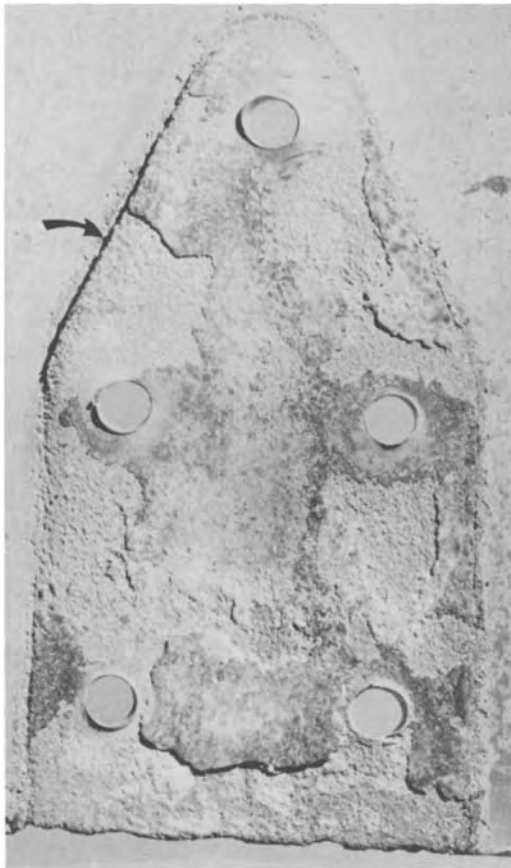
Fig. 4 Typical example of galvanic corrosion combined with crevice corrosion on a 5052-H34 aluminum-alloy engine fan blade that had been riveted between two steel "spiders." The outline of the spider on the engine side of the fan blade is shown by the corrosion products and the pitting that resulted from both galvanic and crevice corrosion from road salt and moisture around the edge of the spider. Bending fatigue fracture originated at pits on other blades and all along the arrowed edge of the spider on this blade.
