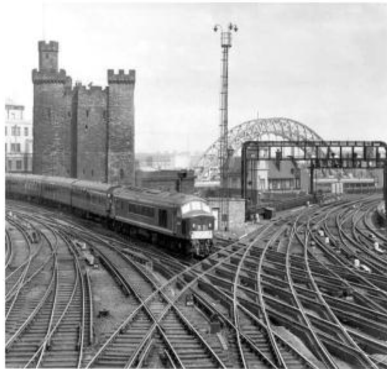
Railway crossing fabricated from manganese steel cast sections
