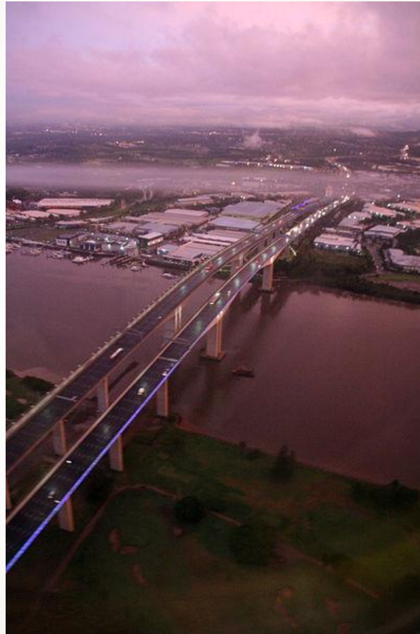
Gate Way Bridge, Brisbane
