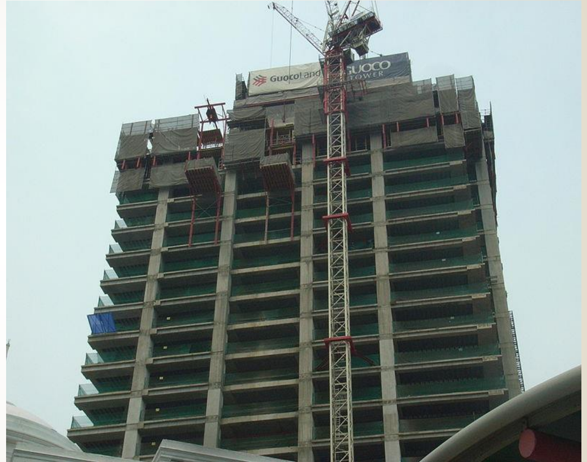
Guoco Tower, Singapore (Under construction)
