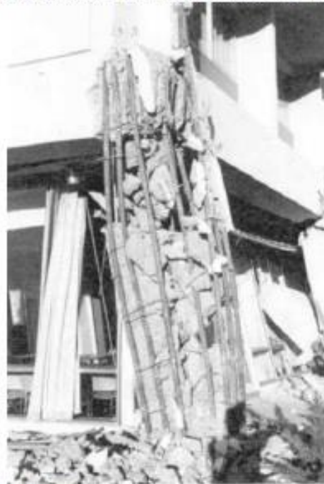
(b) Brittle failure of a reinforced concrete column
