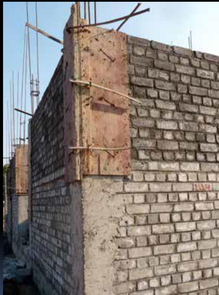
Formwork in place at upper portion of a RC tie-column
