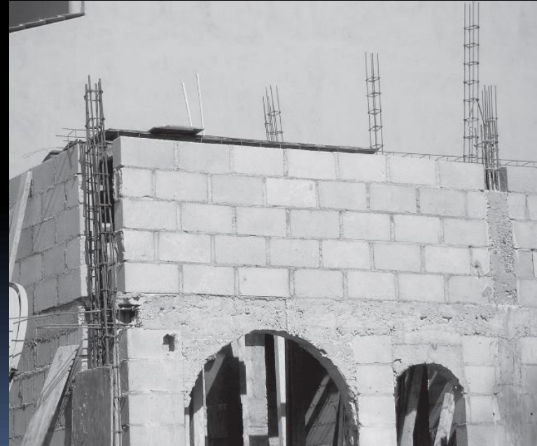
RC frame construction in Cambodia (left) and confined masonry construction in Mexico (right)
