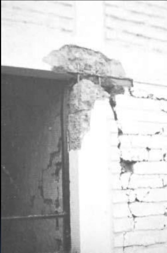
Damage to confined masonry construction in the 1985 Llole, Chile
