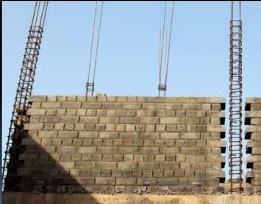
Masonry wall between adjacent tie-columns (construction in progress)
