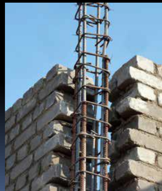
Tothing at the wall-to-tie-column interface
