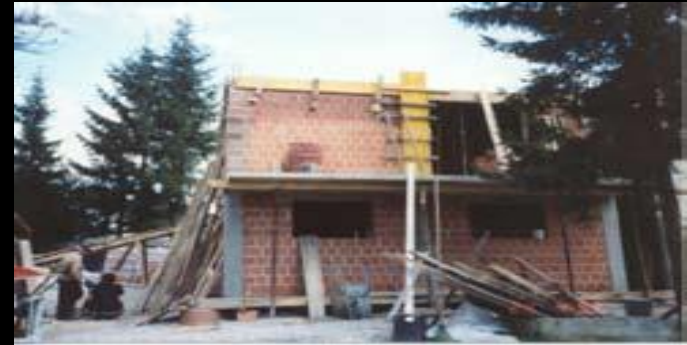
Confined masonry housing during construction in Slovenia
