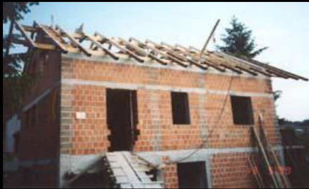
Confined masonry housing during construction in Slovenia
