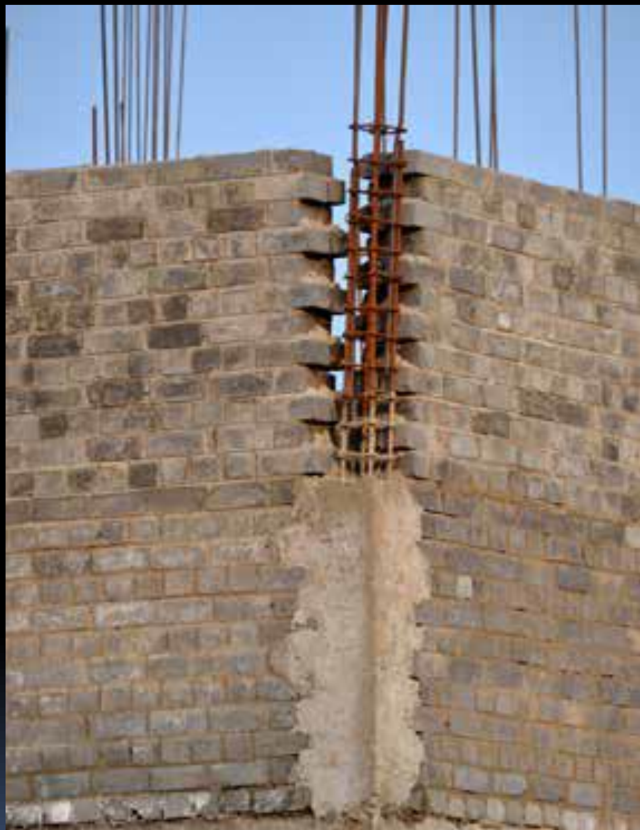
Concrete construction completed at lower portion of a RC tie-column
