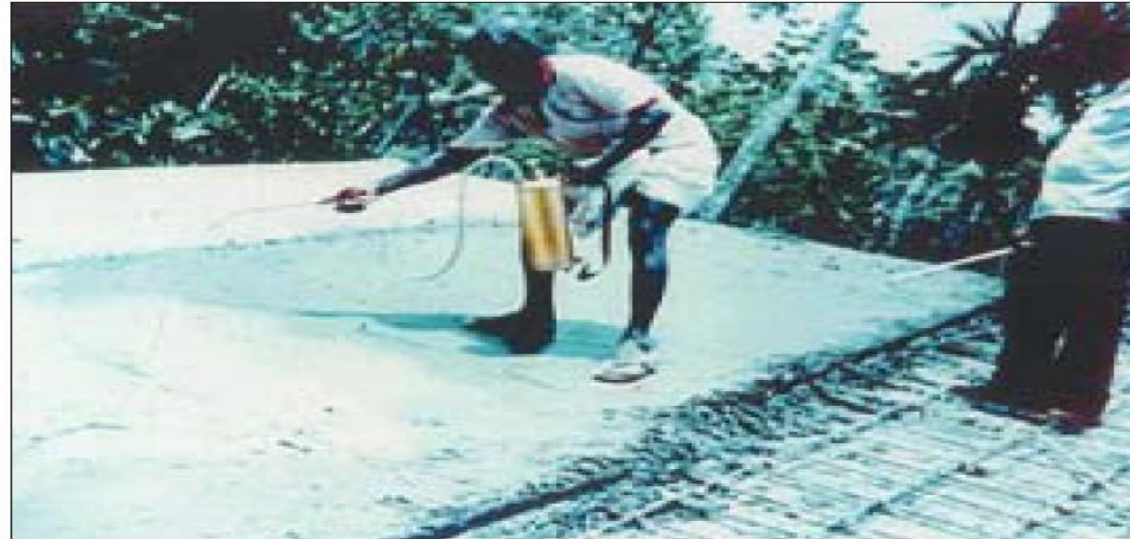
Membrane curing by spraying.
